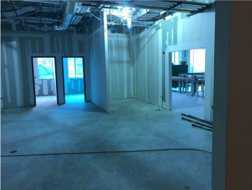
Installation of sheetrock – Level 3
