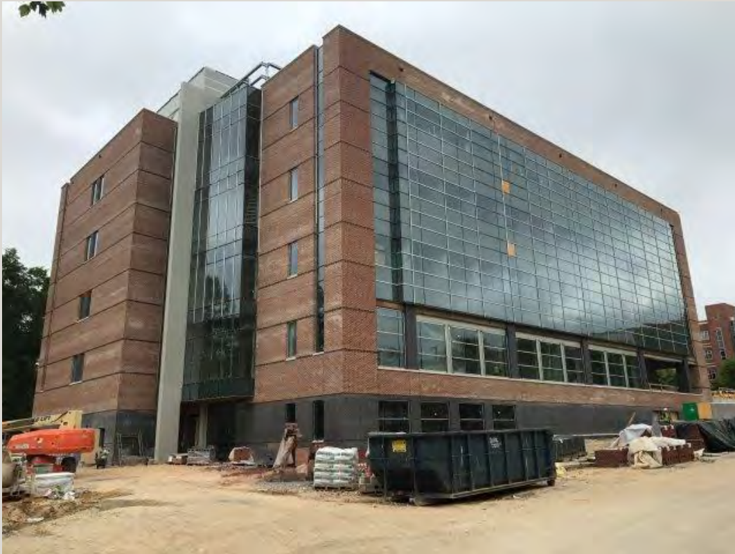
Curtainwall Glass installation
