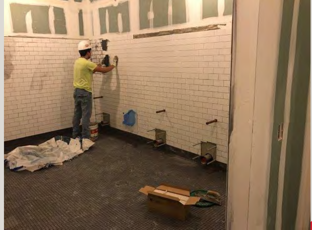
Applying grout to tiles in Toilet – Level 2
