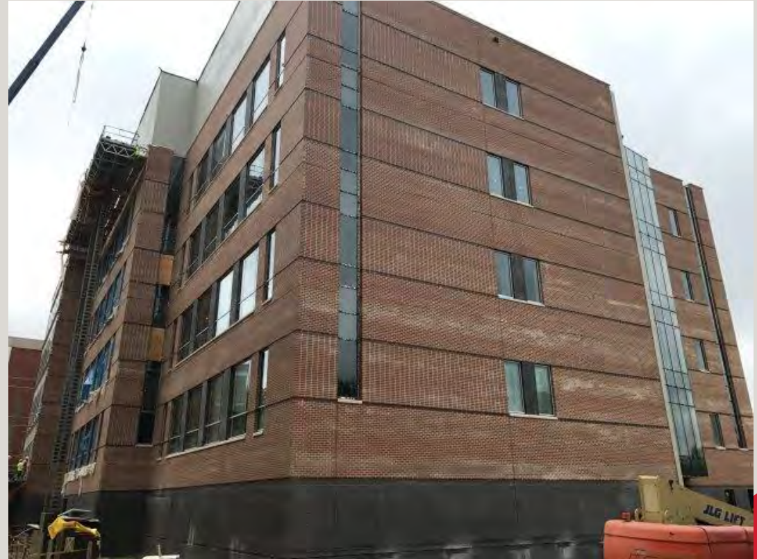
Exterior Masonry Veneer installation
