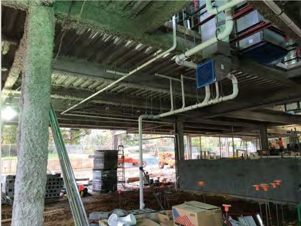
Plumbing pipe installation at restroom
