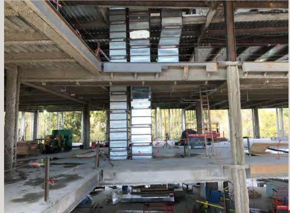
HVAC duct riser installation
