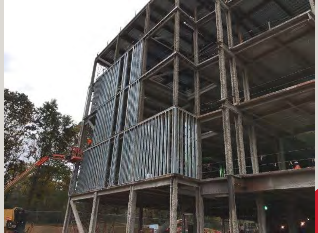
Exterior stud framing installation
