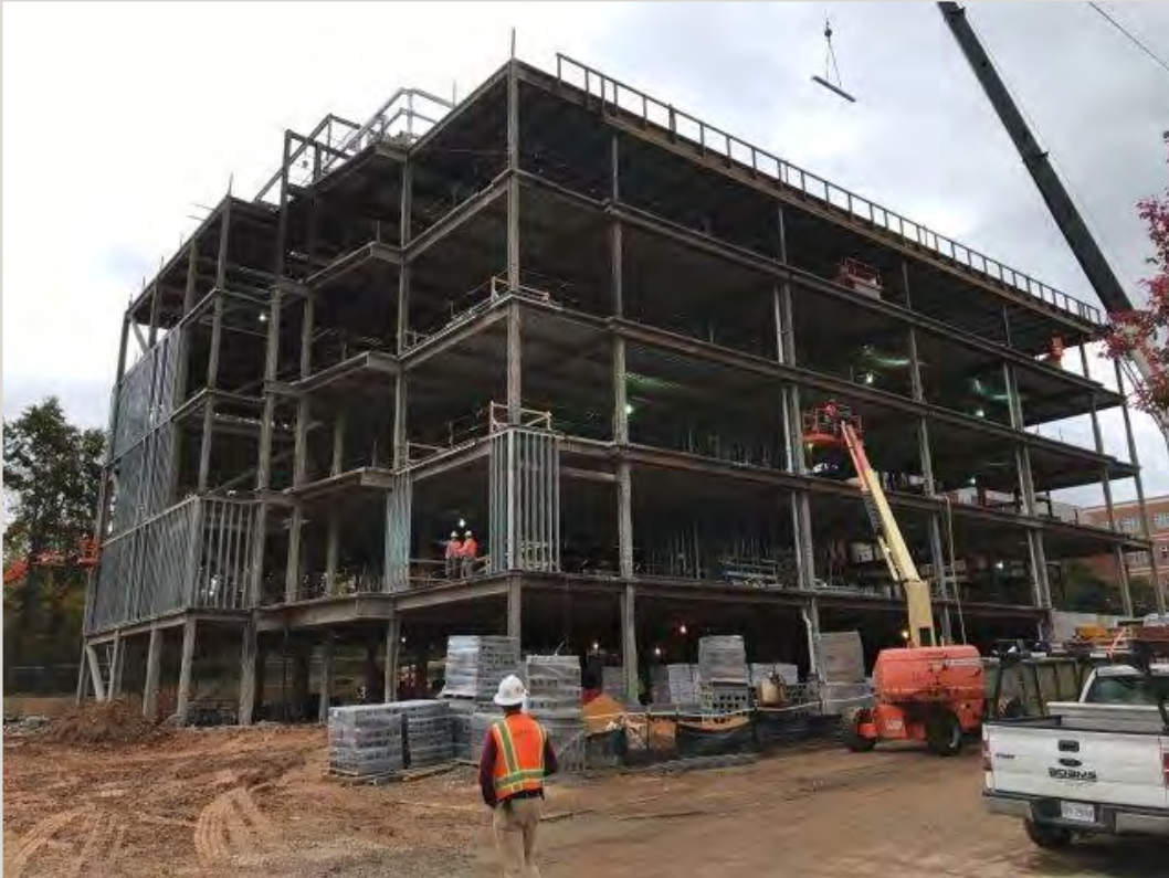
Structural steel frame and stud installation
